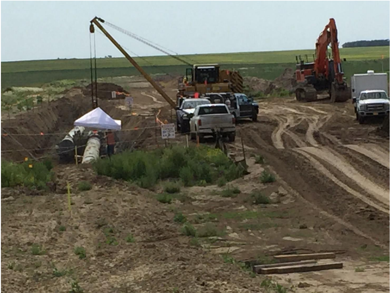
Welding crews welding pigs head onto end of pipe.
