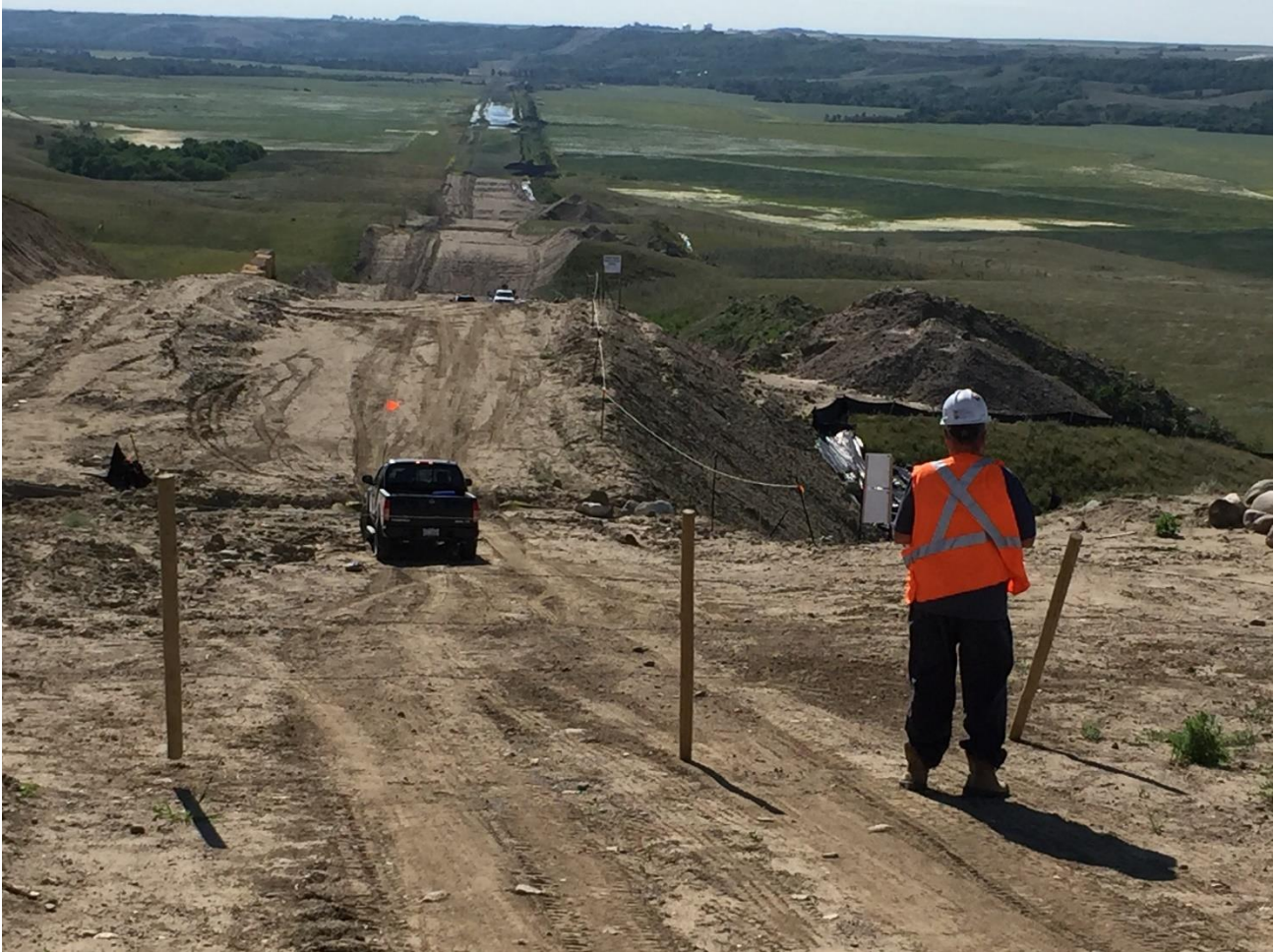
Deficiency crew fixing fence and water breakers at Qu'Appelle valley.
