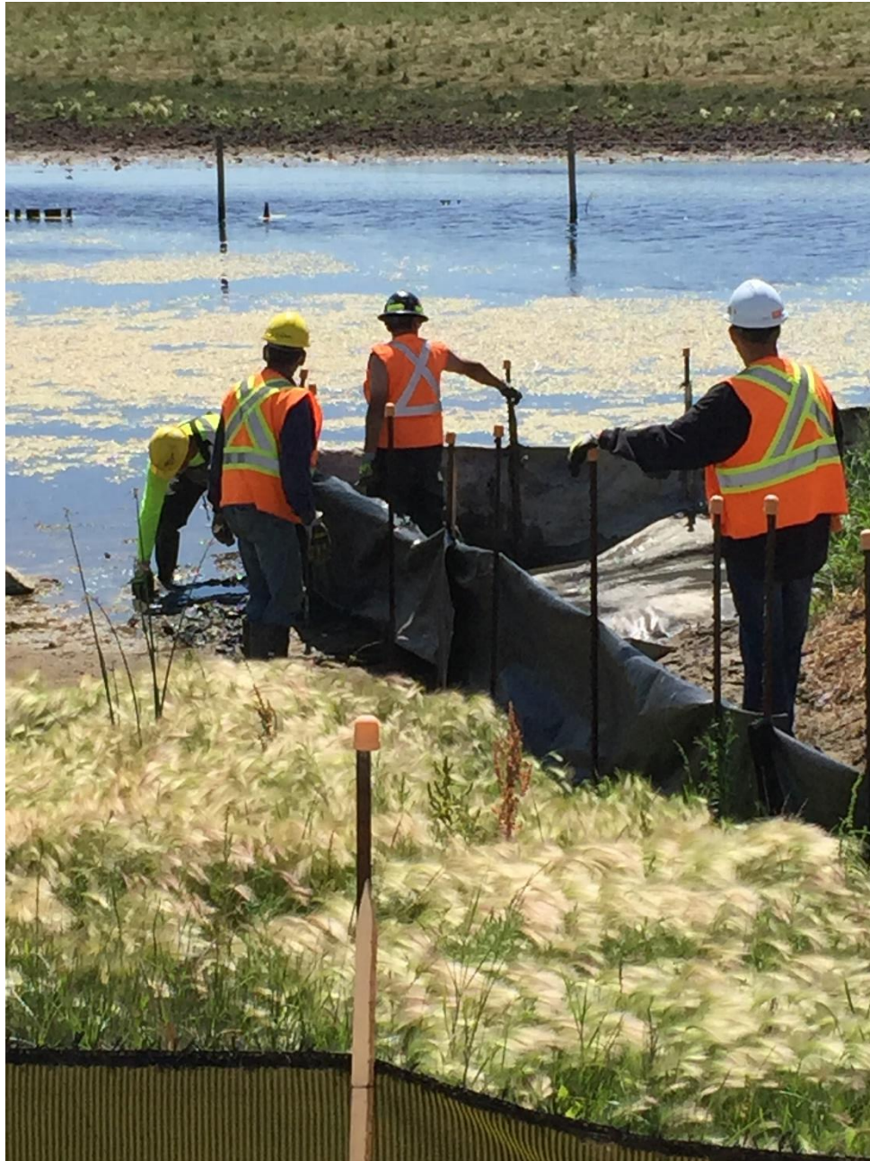
Deficiency crew repairing silt fence at wetlands.
