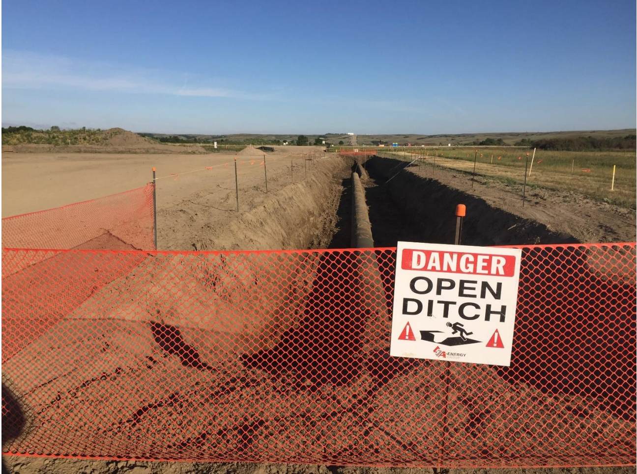
PIPE IS EXPOSED SO THAT IT CAN BE HYDRO TESTED AT A LATER DATE.
